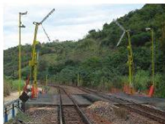
Ore Sprinkler System - Vale
