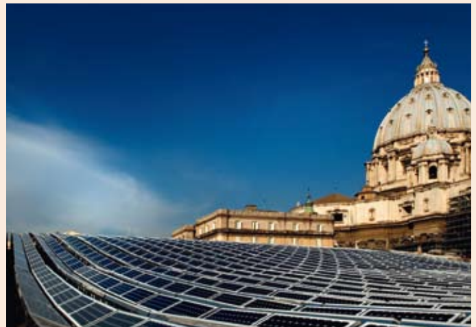
PV installation at the Vatican
